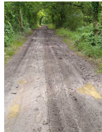
Motor vehicle ruts on the route, July 2021, five years after repairs to remedy ruts and improve the route.
