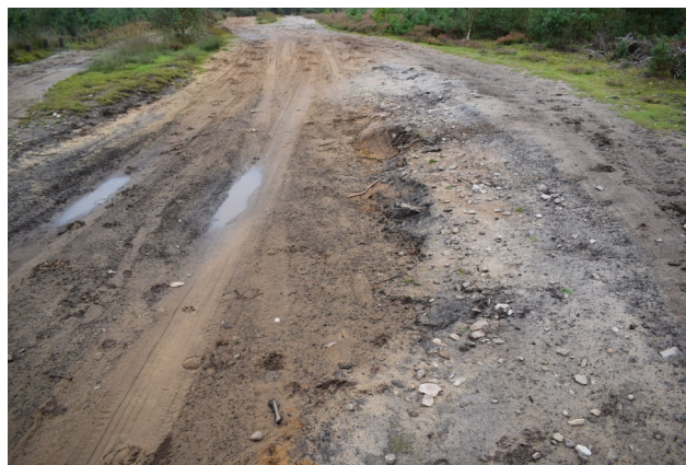
Motor vehicle damage to/widening of Sandy Lane, September 2017. This lane is in the Surrey Hills AONB and is part of a SSSI for its heathland flora and fauna. In its 2022 publication on green lane management LARA claims that voluntary restraint, stumping to reduce the width/deter off-lane driving and a night-time TRO would be sufficient to remedy the damage to the surface of this lane and adjacent land.
